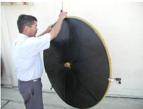
USE CLAMPS TO HOLD ASSEMBLED SHIELD TO WHEEL FRAME
